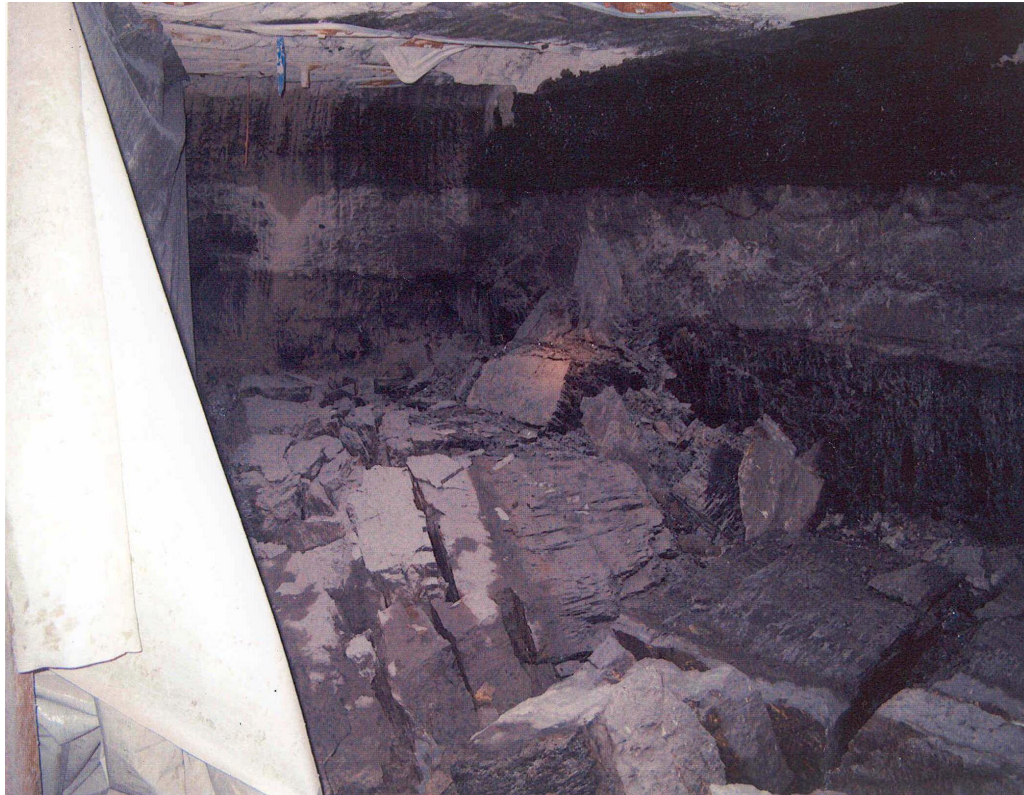
Figure 29 This photo was given to me by the mine head—it shows a rib roll that happened earlier in a different part of Deep Mine 36. The thick chunks of coal and rock peeled off the mine wall to the right and tumbled to the ground, like a slice of cake plopping down when it's cut. The plastic sheet to the left is a curtain, used to control air flow in the mines. The strata of rock and coal are apparent in the mine wall. Photo courtesy of Mike.
