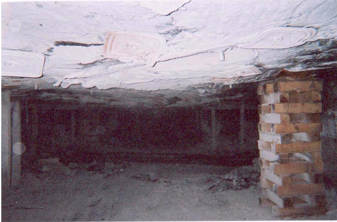
Figure 43 A crib to the right and timbers support the buckling “bad top” mine roof. The ceiling here “bellies down” and sags in the middle under the weight of the mountain. Photo by the author.
