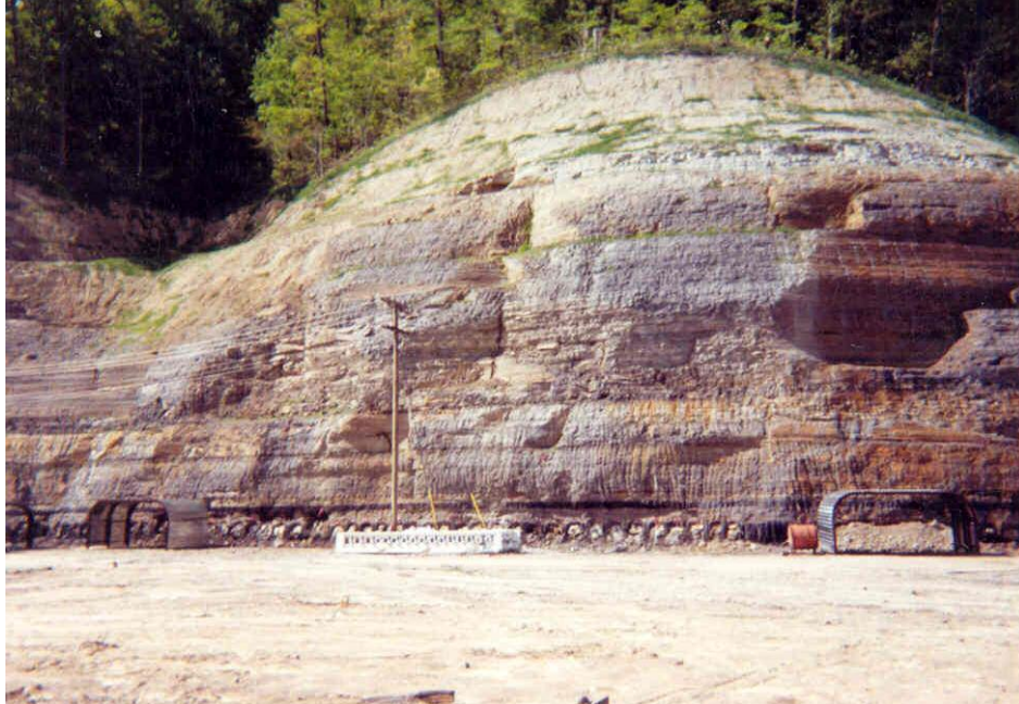
Figure 45 The mountainside before cutting in to form the drift mouth. Photo courtesy of Mike.
