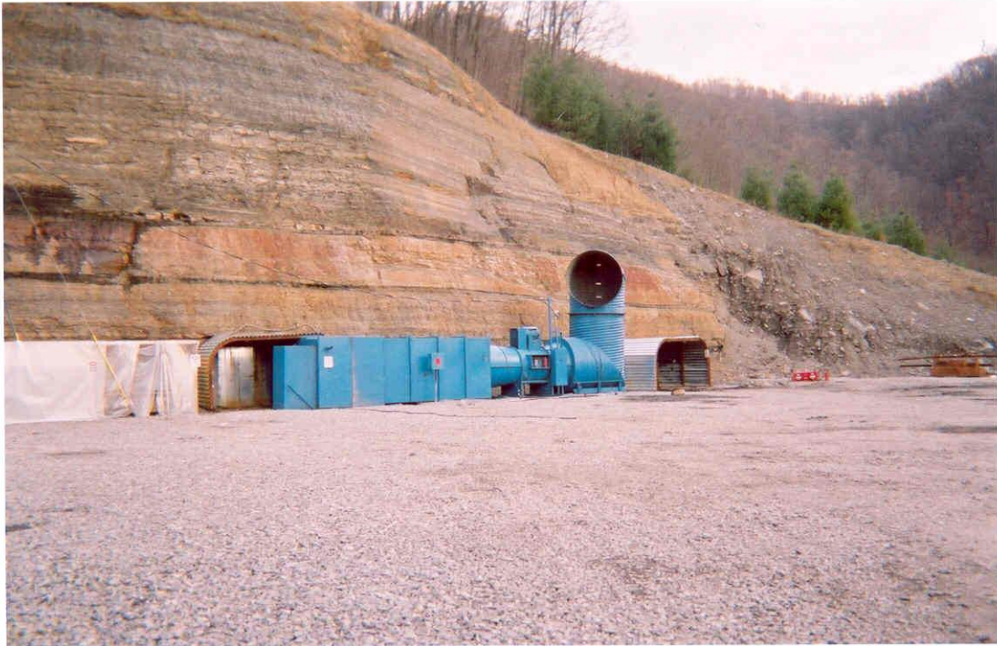
Figure 25 Ventilation fan and large duct connecting fan to the interior of the mines. Photo courtesy of Mike.
