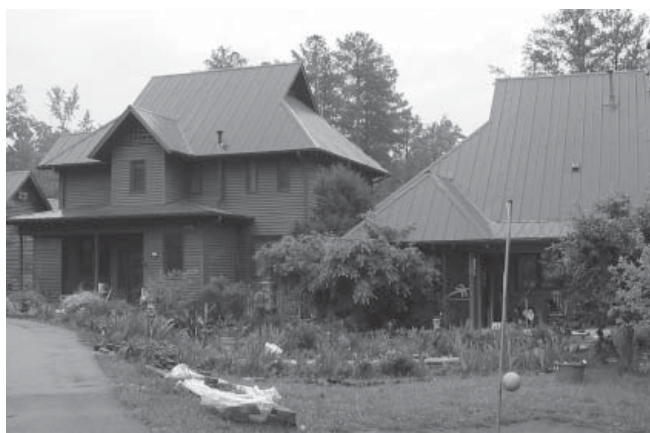
Arcadia community homes feature a variety of designs with green building elements. Photo by Rawley Vaughan.
