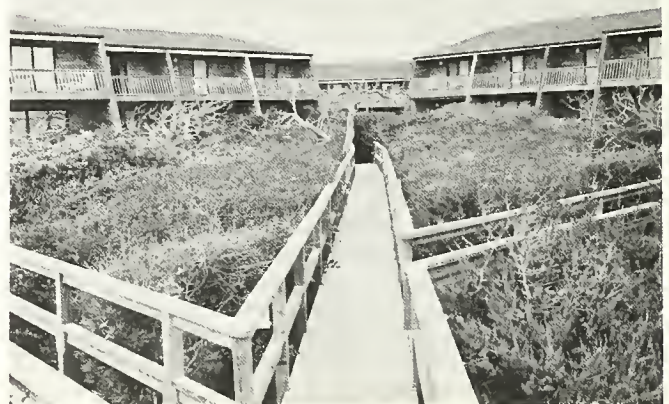
Figure 6. Elevated boardwalks beneath canopy limit disturbance of the maritime forest. Photo by L. Zucchini
