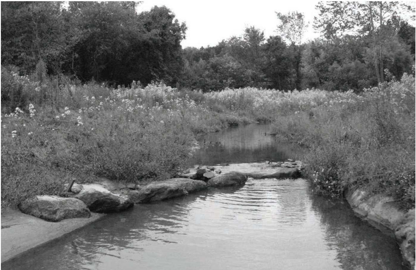
Valley Fields Farm Stream Restoration, Davidson County, N.C.: Post-construction example of similar restoration project (Rock Cross Vane). Photo courtesy of Kimley-Horn and Associates, Inc.
