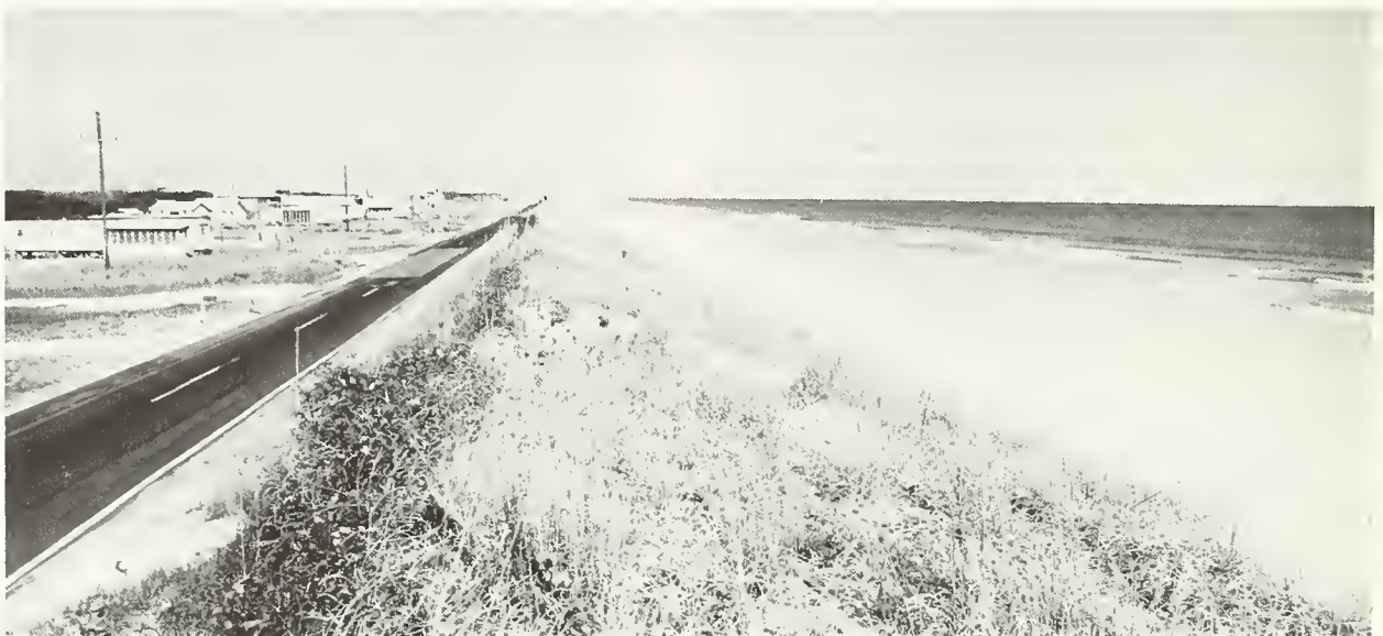
Roads constructed too near the shoreline tend to disrupt natural barrier island processes
