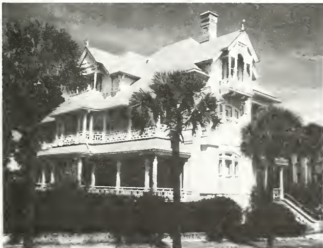
Double gallery porch design provides summertime energy efficiency.
