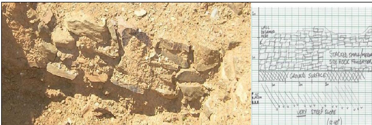
**Figure 4-10.** Stacked stone masonry wall, photo with field map in profile
