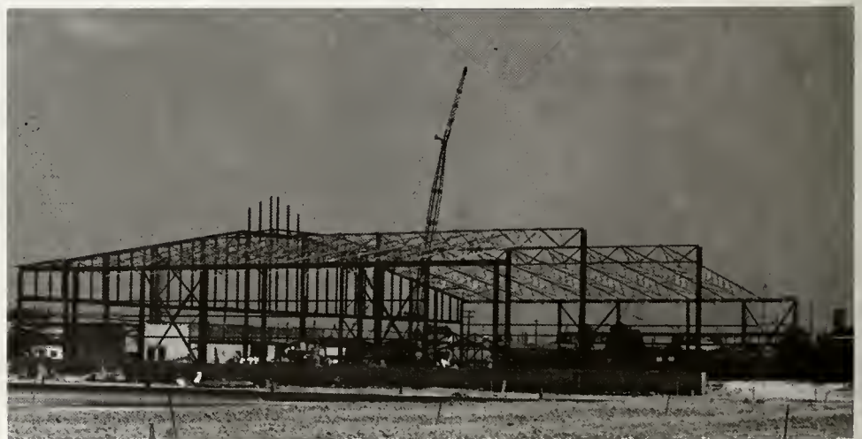
New transit shed and paved storage area under construction at the Port of Tampa.
