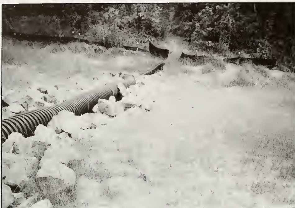
Good practice: A slope drain, anchored in rip-rap, channels run-off to where it won't erode the slope.
