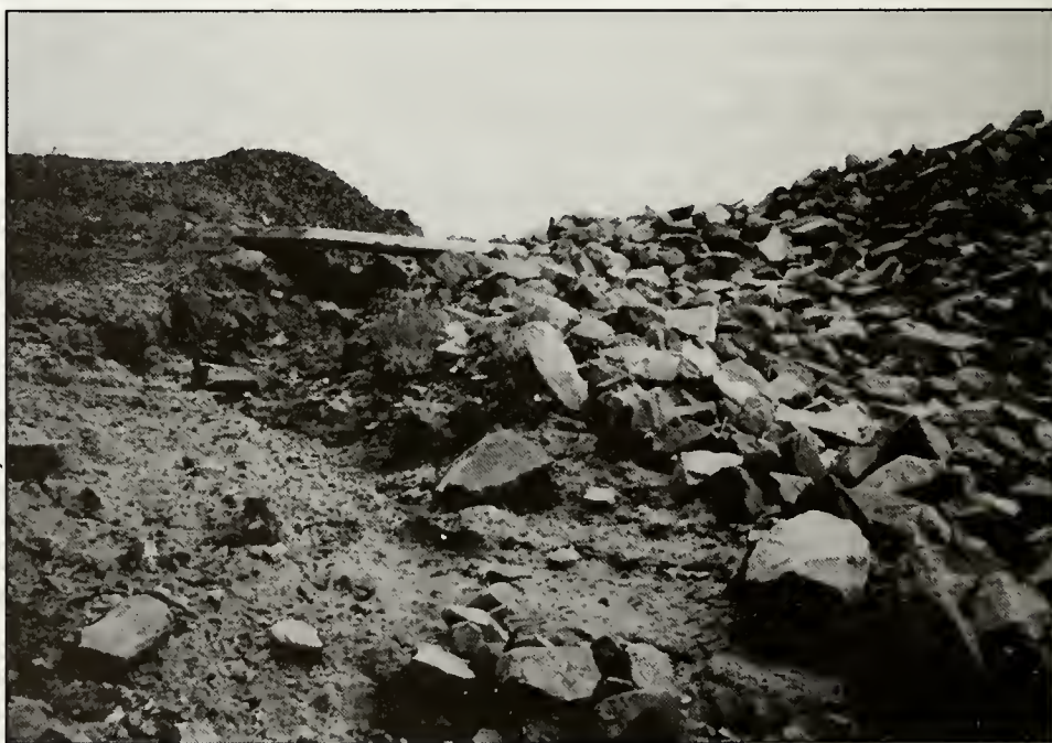
Bad practice: A rip-rap channel, designed to filter out sediment, is ineffective because a trap failed, allowing water to bypass it.
