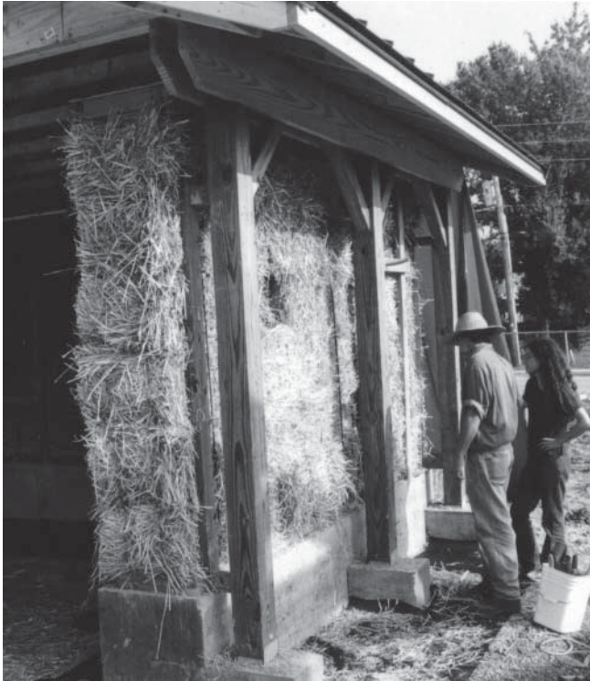
Figure 1. Example of straw-bale construction used in the Berea College Eco-village in Berea, Kentucky. Photo courtesy of Ann Hartell.
