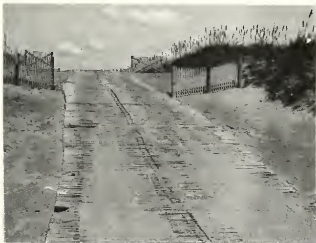
Figure 4. Using wooden or aluminum crossover mats can reduce the impact of vehicles on the dunes.
