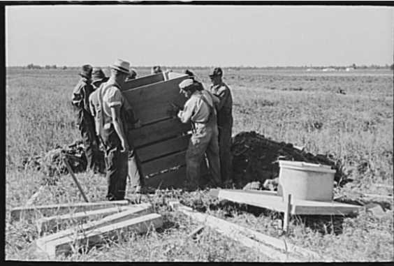
Figure 2: "Privy erection. Placing wood cribbing in privy well."
