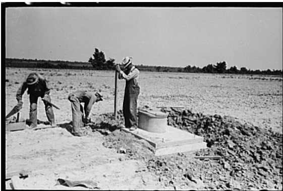
Figure 3: "Privy erection. Back filling and tamping the earth around sanitary base and mud sill."
