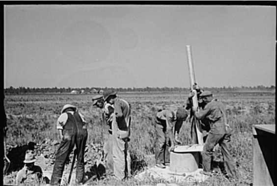
Figure 4: "Privy erection. Fitting vent stack and lid on sanitary well."
