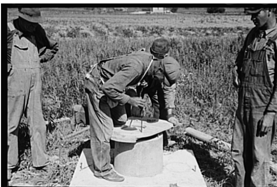
Figure 5: "Fitting seat and lid on sanitary base of privy."
