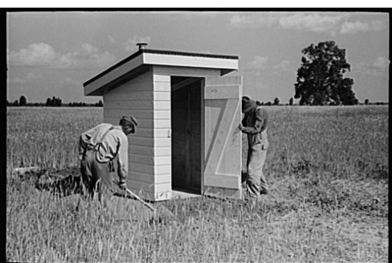
Figure 6: "Final operation in setting of sanitary privy at the job site."
