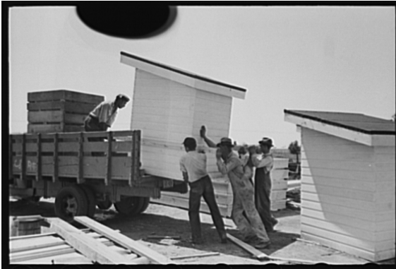
Figure 1: "Loading completed privy houses on truck for delivery to site."
