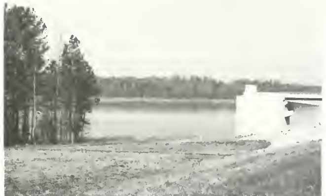
The Dam at Falls of the Neuse Reservoir.
