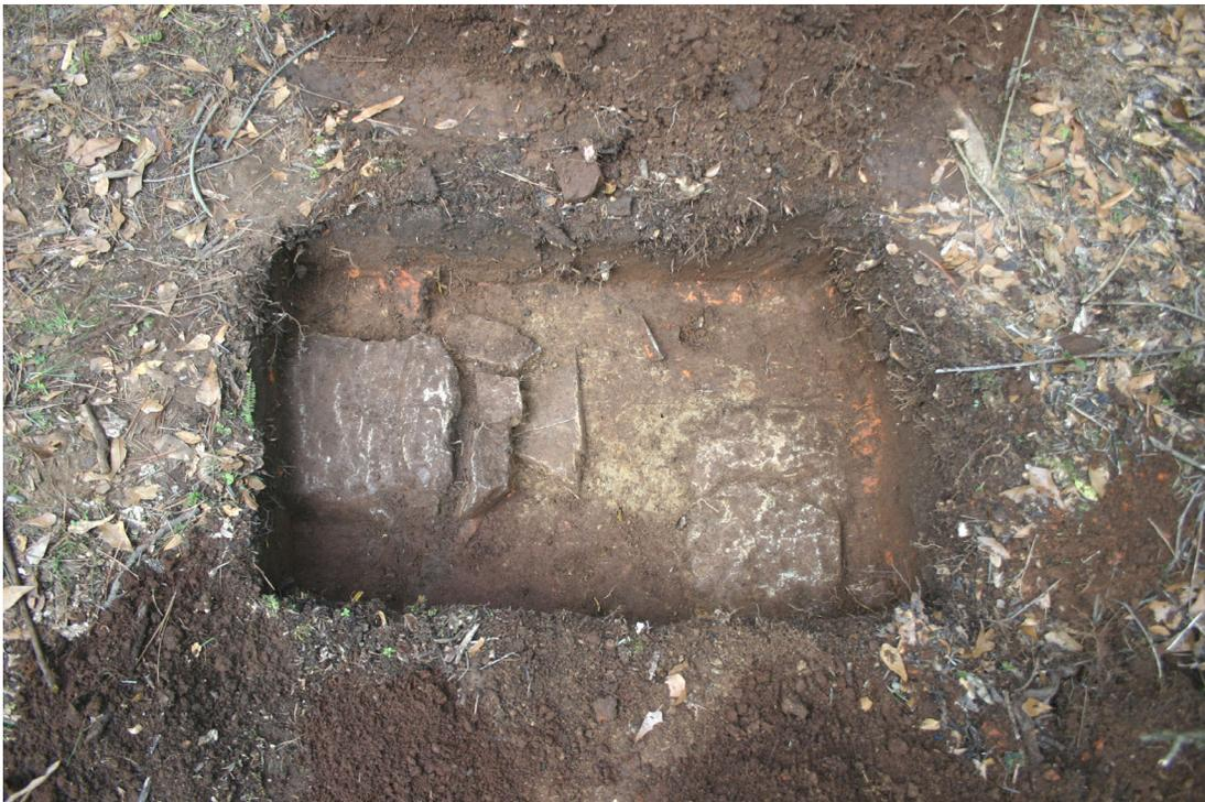
Figure 17. Top of stone foundation in Test Unit C. Note the brick rubble along the top and right edges, the dark fill along the interior side of the wall, and the sand mortar between the stones. View to north.
