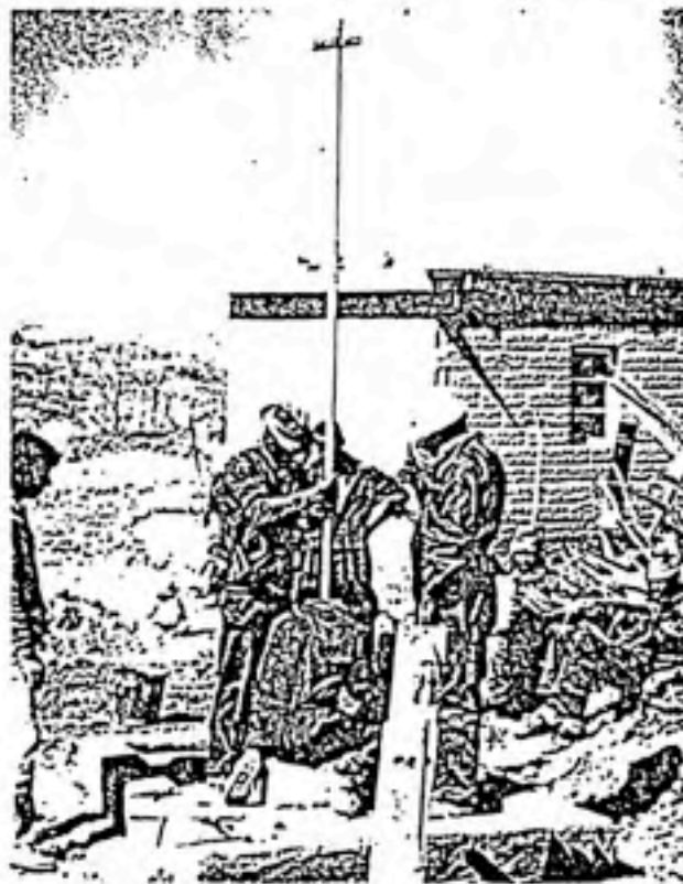
The Consallen's plastic drop pipe makes installation and removal of the underground equipment a simple operation (above). The completed installation (below) is the closest currently available to the lift panel's VLDiff pump head.
