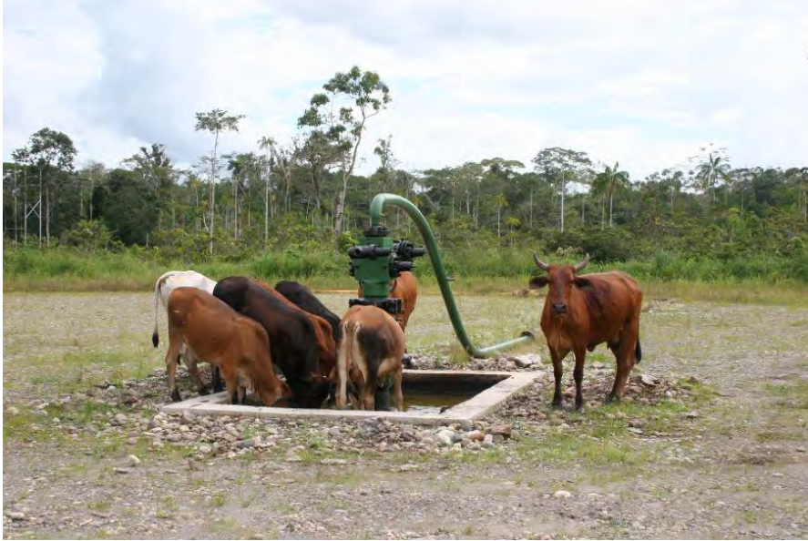
Figure 7 A wellhead of a reinjection well. Reinjection wells are painted green, live wells are painted red. Livestock are often attracted to the salty water that accumulates in the containing box [cubeto] around the well head. Source: Manuel Pallares.
