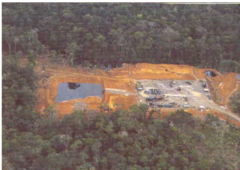
Figure 2 Well Platform and pits. To the right the platform is visible, with the access road leading off the right hand corner. The well is located in the center of the platform. One waste pit is visible to the left of the platform as well as a smaller pit off the upper right-hand corner of the platform. Source: Manuel Pallares.
