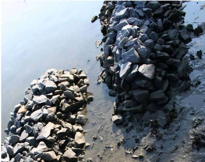
Figure 4.A2. Photo of a sill with a) drop-downs and b) gaps between the sill structures. Both designs were sampled in this study. Photos were taken on the flood tide at approximately 3 hours before high tide for (a) and 5 hours before high tide for (b).
