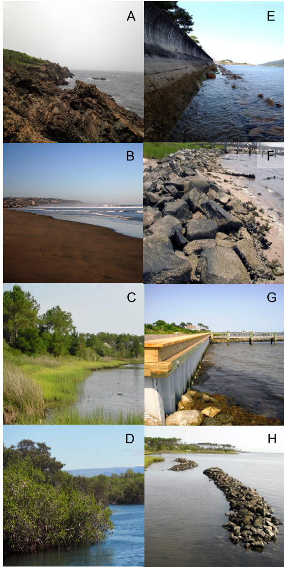
Figure 2.1. Types of natural and artificially hardened shorelines found in the United States: a) rocky shore; b) beach; c) tidal marsh; d) mangrove; e) sea wall; f) riprap revetment; g) bulkhead; and h) breakwater. For images of other shoreline types found in the U.S., refer to the NOAA ESI shoreline types image gallery ( http://response.restoration.noaa.gov/esi-shoreline-types ).
