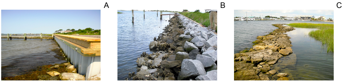
Figure 3.1. Photographs of shoreline types: a) a bulkhead: a vertical structure typically constructed of vinyl composite, concrete, asbestos, or treated wood placed at or above the observed high water mark; b) a riprap revetment: a sloped structure typically constructed of granite, marl, or concrete placed at or above OHWM; and c) a sill: a structure typically constructed of granite, marl, or oyster shell, seaward of marsh.
