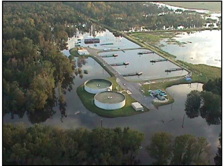
Figure 2: Peachtree Wastewater Treatment flooded after Hurricane Floyd. Source: City of Kinston, NC
