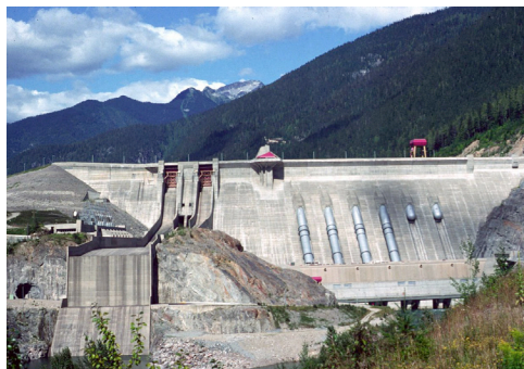
Figure 2-8. Dam on Columbia River, British Columbia. Turbines in face of dam.
