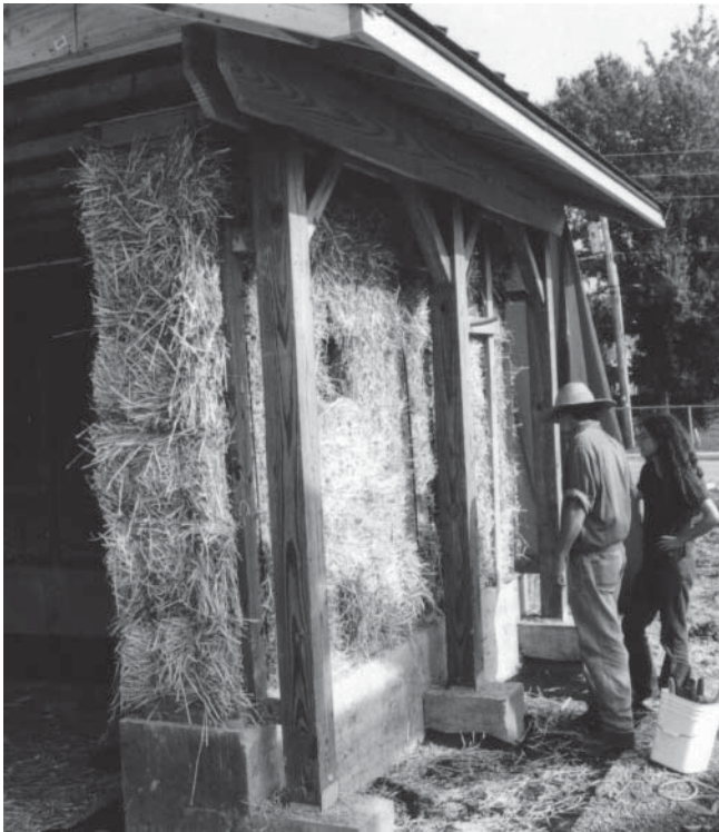
Figure 1. Example of straw-bale construction used in the Berea College Eco-village in Berea, Kentucky.
