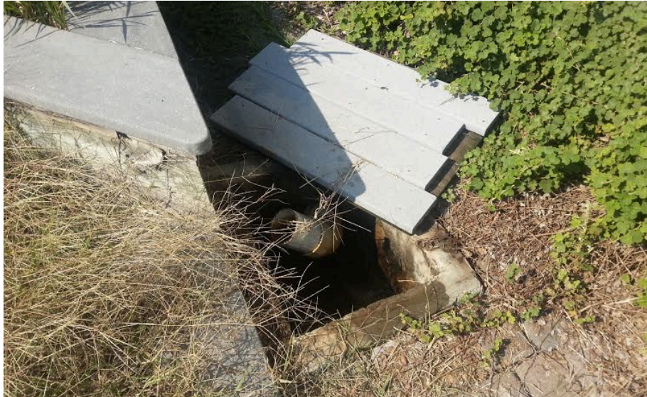
Figure 7. Distribution box containing source water
