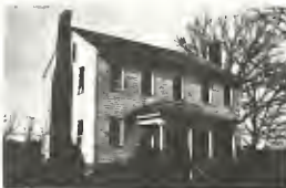
FULEWIDER-CARPENTER HOUSE Catawba County
