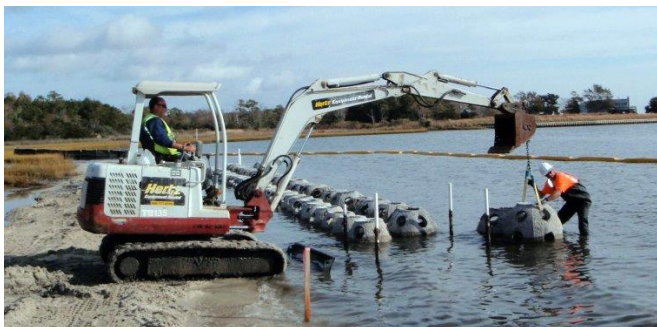
Figure 8-1. A contractor places the domes into the sound as part of a project in 2011.
